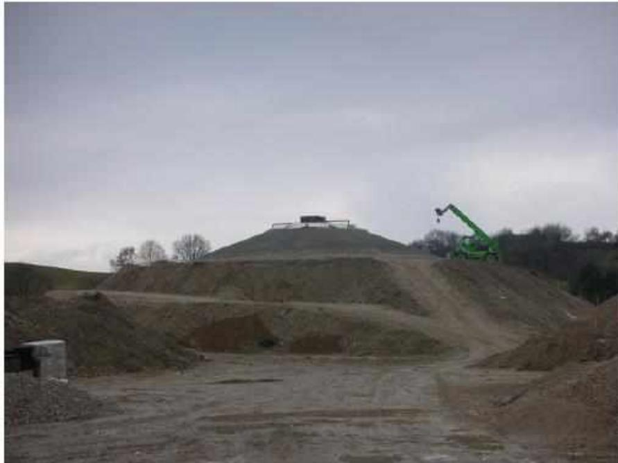
Figure: Sand layer at above ground TTES system
