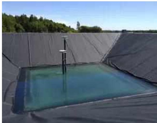
Figure 3:10 Pit of PTES system without cap [11]
