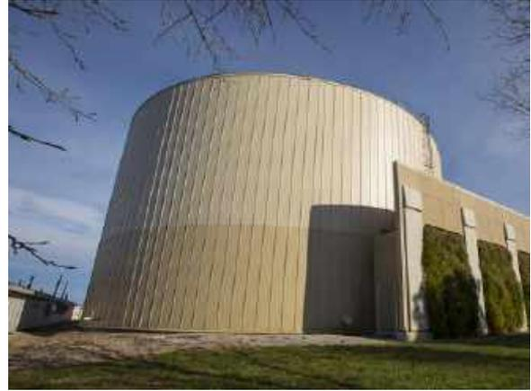
Figure 3-7: partially dug-in water storage tank (Solites)
