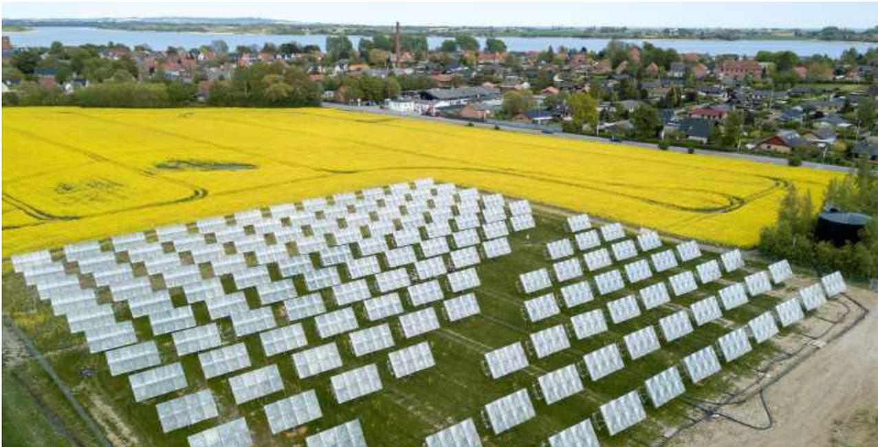
Figure 3- Large scale concentrating collector field as part of a district heating network.
